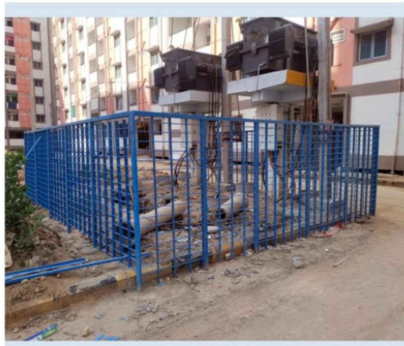
2BHK GOVT APARTMENTS THUMUKUNTA
